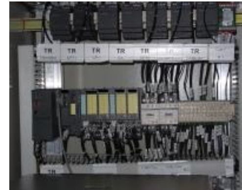
Cabinet containing a safety controller and the SIL 3 program
